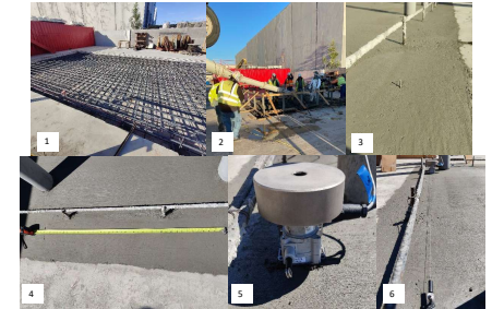
Different steps involved in String Potentiometer Test
